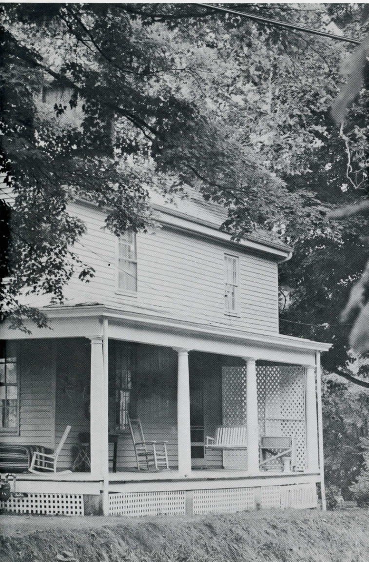
(left) Lemuel Chenoweth home built in 1847 overlooking the Tygart River and next to his covered bridge (below) which has been demolished. The house is on the old Staunton-Parkersburg Turnpike.
