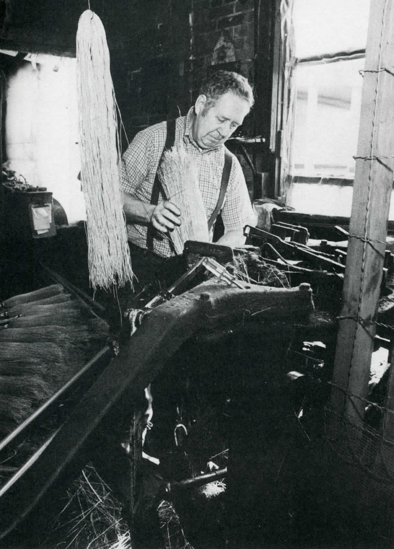
Left: Jim Shaffer sews a broom on a Baltimore sewer, one of the factory's two sewing machines. The next step is to trim the end of the broom.
