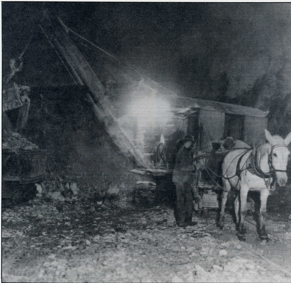
Mules provided the motive power for limestone mining for much of the quarry's history. Cars of stone were taken to the kilns, for "burning" into lime. Photographer unknown, about 1920.
