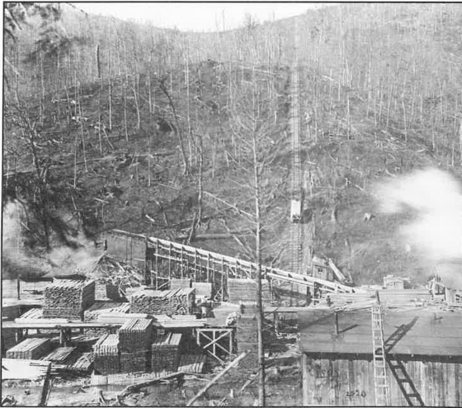
The rail incline at Braucher was an over-the-mountain affair. The photograph above shows the sawmill side in Mountain Lick Valley, with a load of lumber heading uphill. The other picture shows the other side, where loads came down to the Western Maryland Railway tracks. Just visible at the top is an installation consisting of an engine house and operator's residence. Photographer unknown, about 1909; courtesy Mrs. G. E. Hevener and Pocahontas County Historical Society.
