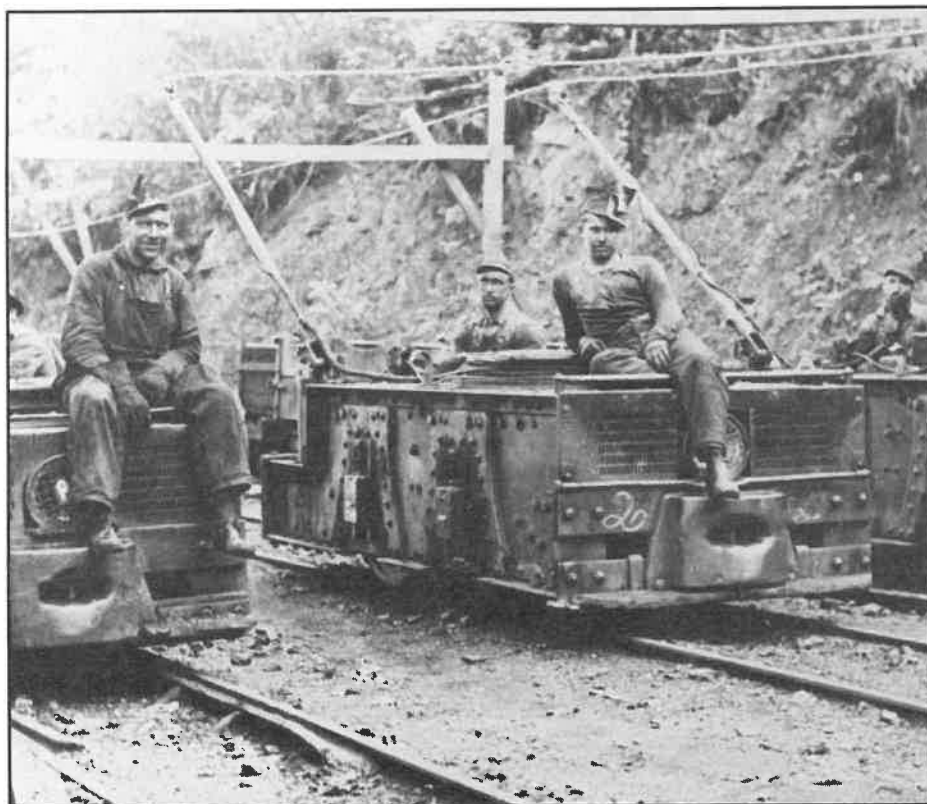
Mine electrification, introduced at Gauley Mountain soon after Garland Skaggs began work there, offered a lifelong career opportunity for working with the new technology. These mine motors draw power from the trolley wires overhead. Postcard view, date unknown; courtesy Gladys Skaggs Brown.
