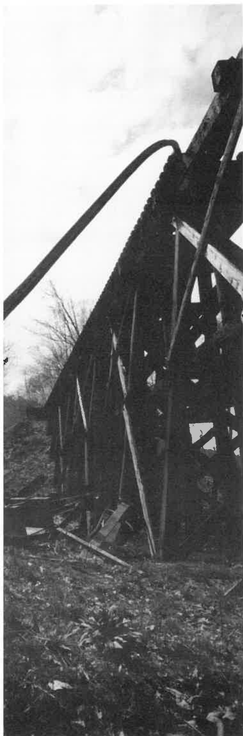
The power of the 1985 flood is attested by the twisted steel rails shown in the photo at left. The central span of the railroad bridge into the Trough was lost, as shown above.
