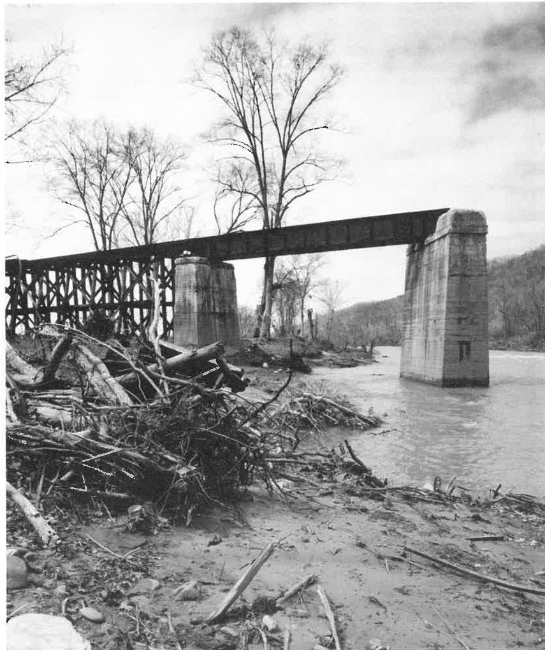
The power of the 1985 flood is attested by the twisted steel rails shown in the photo at left. The central span of the railroad bridge into the Trough was lost, as shown above.
