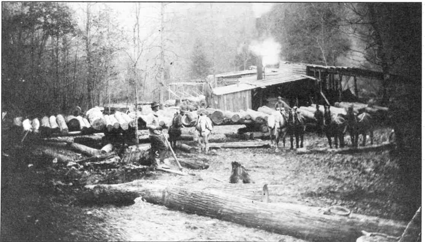
Below: Lloyd Spencer and Hickman owned this steam-powered portable sawmill. This set-up was typical of the early years of the century. Photographer and date unknown.
