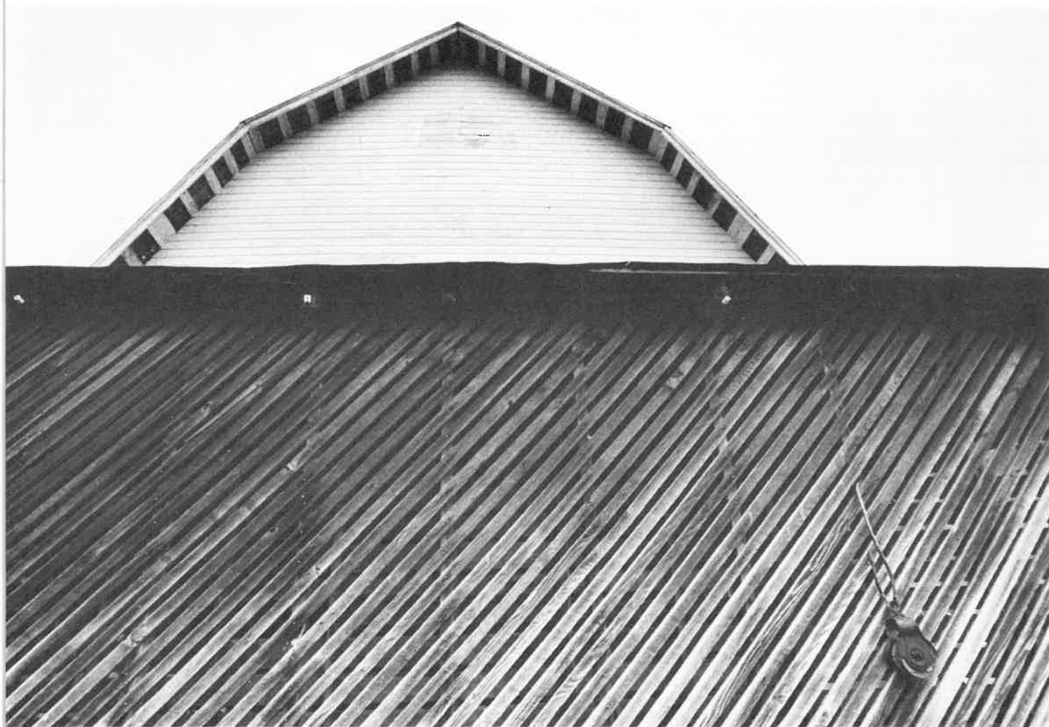
Diagonal siding was best, according to Kimbrew, for its strength and good water run-off. This crib adjoins a Kimbrew barn.
