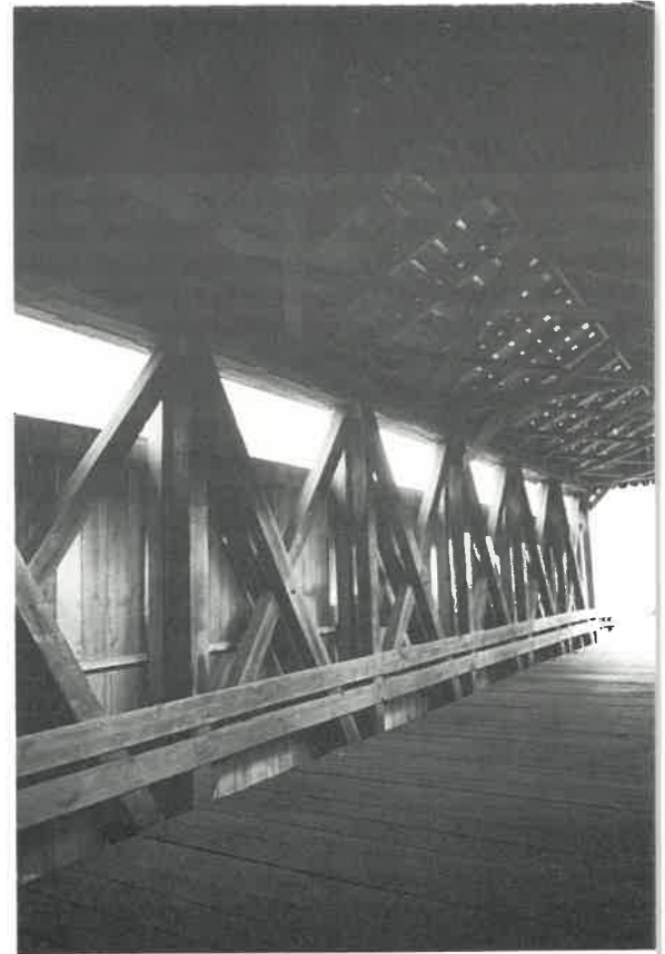
West Virginia's covered bridges generally used a truss or arch-truss framing system. The Barrackville Bridge (above) features a Burr arch-truss, which incorporates a timber arch into a truss framework. The Staats Mill Bridge (right) employs a Long truss, characterized by X-shaped cross bracing.
