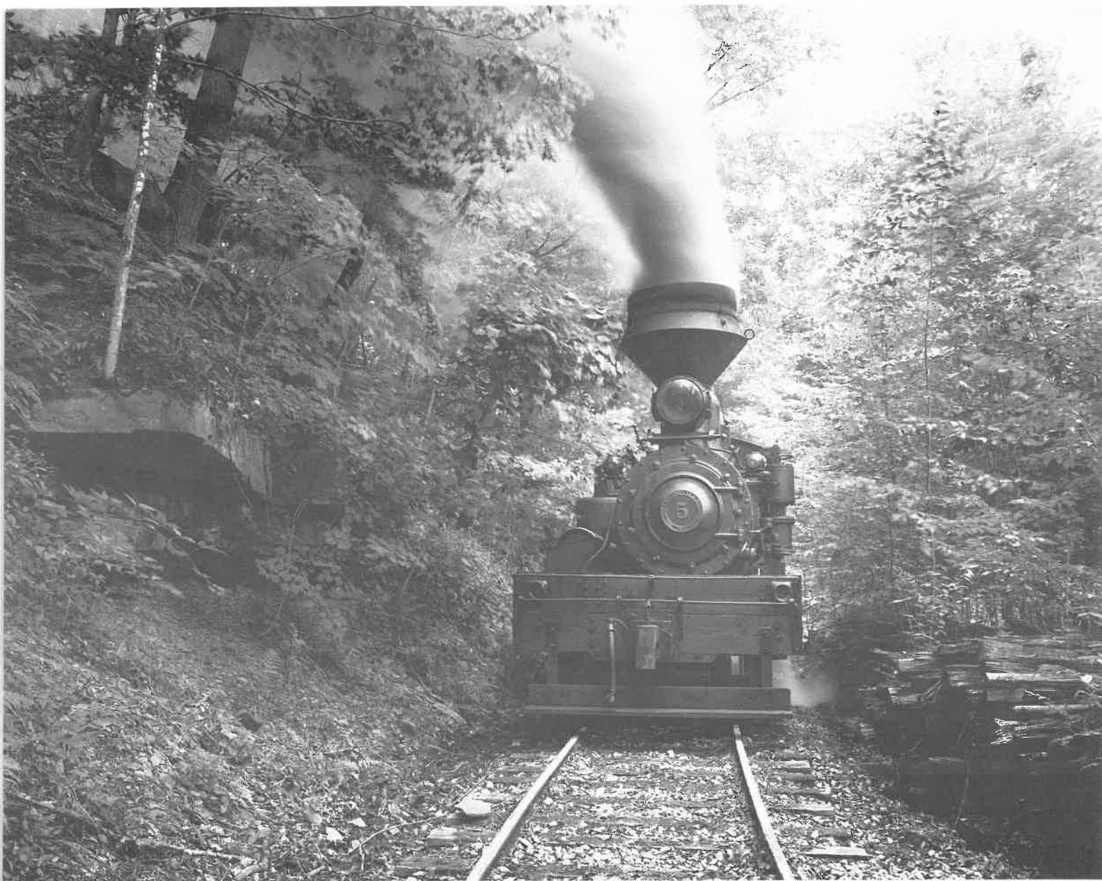
Above: Ted Burdette was the first engineer to put Shay No. 5 on top of Bald Knob, and it remains a family favorite. The off-center boiler on the Shays allows room for the gearing. Photo by Ron Snow, 1985; courtesy State Department of Commerce.
