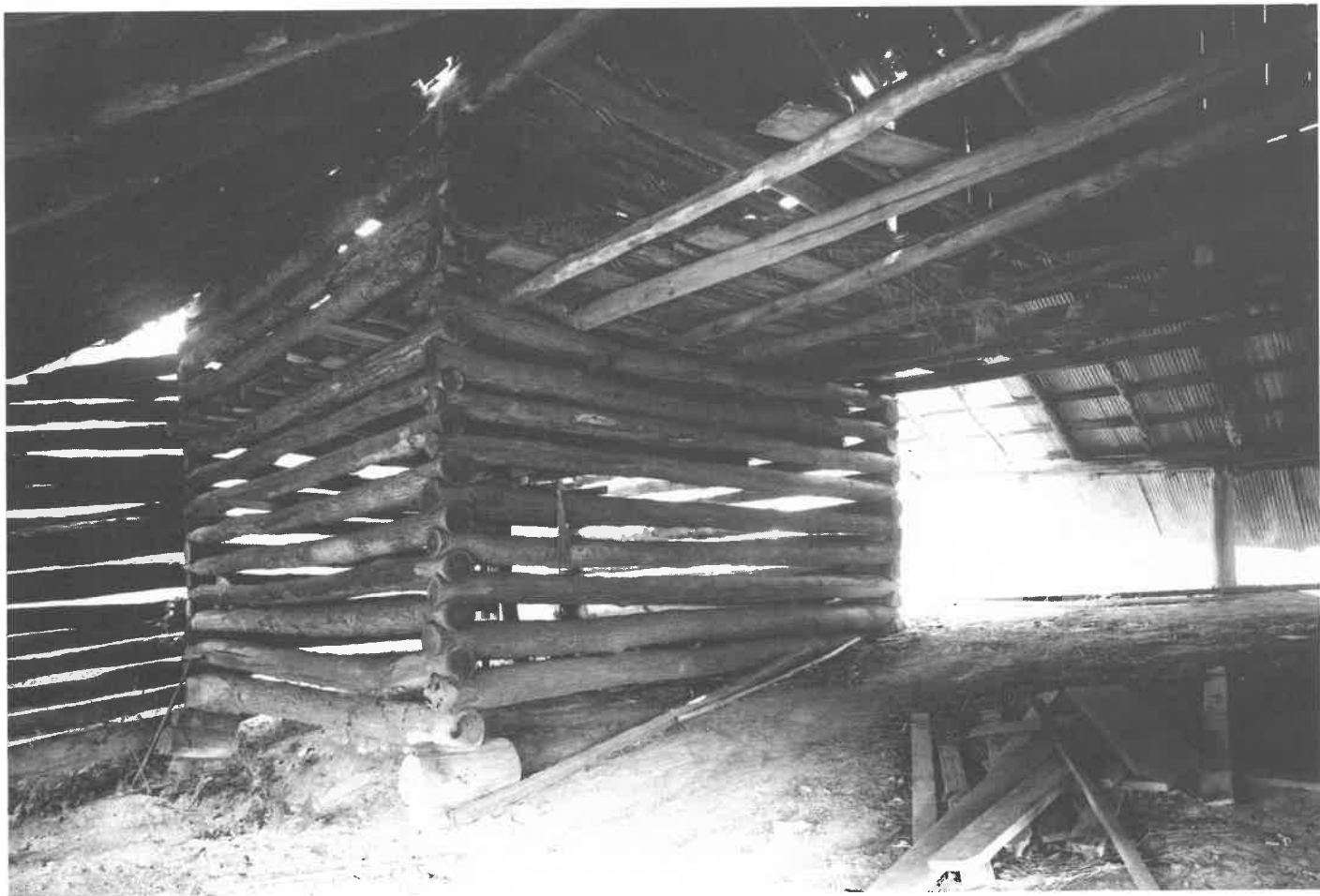
This log barn has stood on the Cottrell place since early in the century. This is a classic "double-pen" design, with one of the log pens shown in the interior photograph. The bottoms of the two pens were used as livestock stalls, and the open breezeway between them offered easy access to the building. Sylvia says the barn was hung full of curing tobacco in season.
