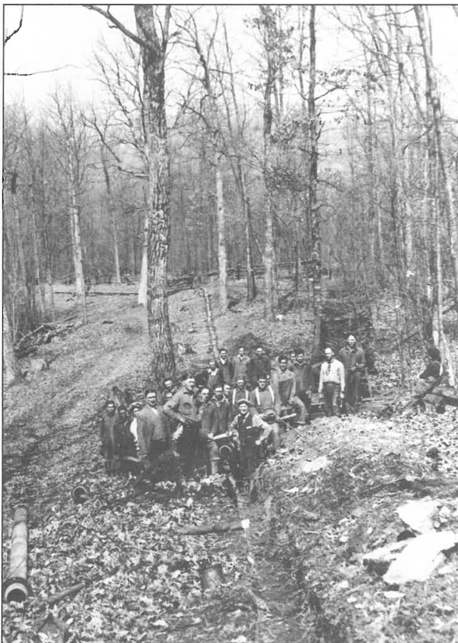
Photographer Perry Cox captured this pipeline crew at work in southeastern Ritchie County. This is from the era of Mr. Sutton's memory, although the date and exact location are unknown.
