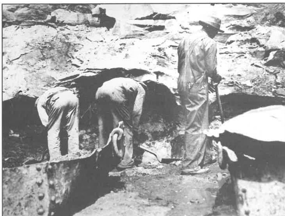
Top: The view from the tunnel, August 24, 1930. This is the downstream portal, nearest Gauley Bridge. Photographer unknown, courtesy State Archives.
