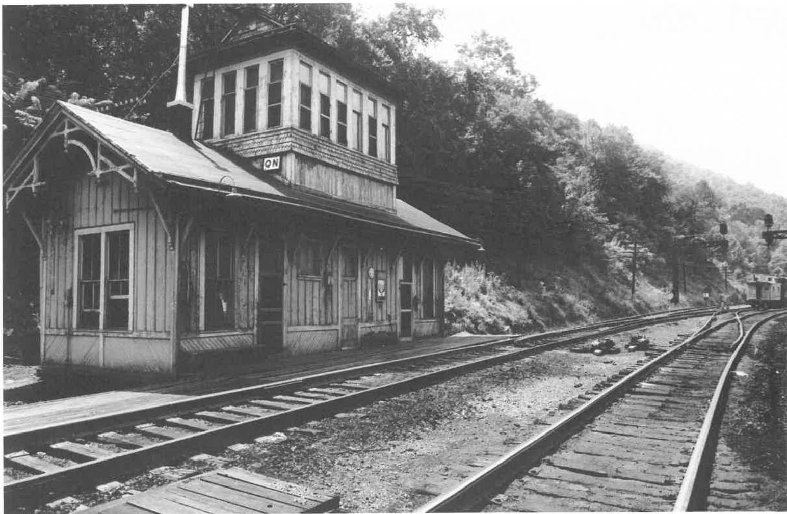
The Quinnimont signal tower — QN cabin in railroad parlance — was a local landmark until demolished by the C&O a few years ago. This photo by Doug Chadwick is from the late 1970's.
