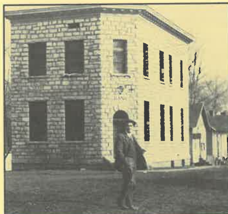
The Bank of Glen Jean is among National Register properties included in the new book of Fayette County historic sites. Photo by William Trevey, before 1917.
