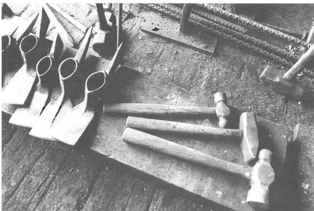
Heat, skill—and good, heavy hammers—were the essence of the tempering process. J.R. Dillon of Raleigh County used these hammers to temper the mattock blades at left. Photo by Doug Chadwick.
