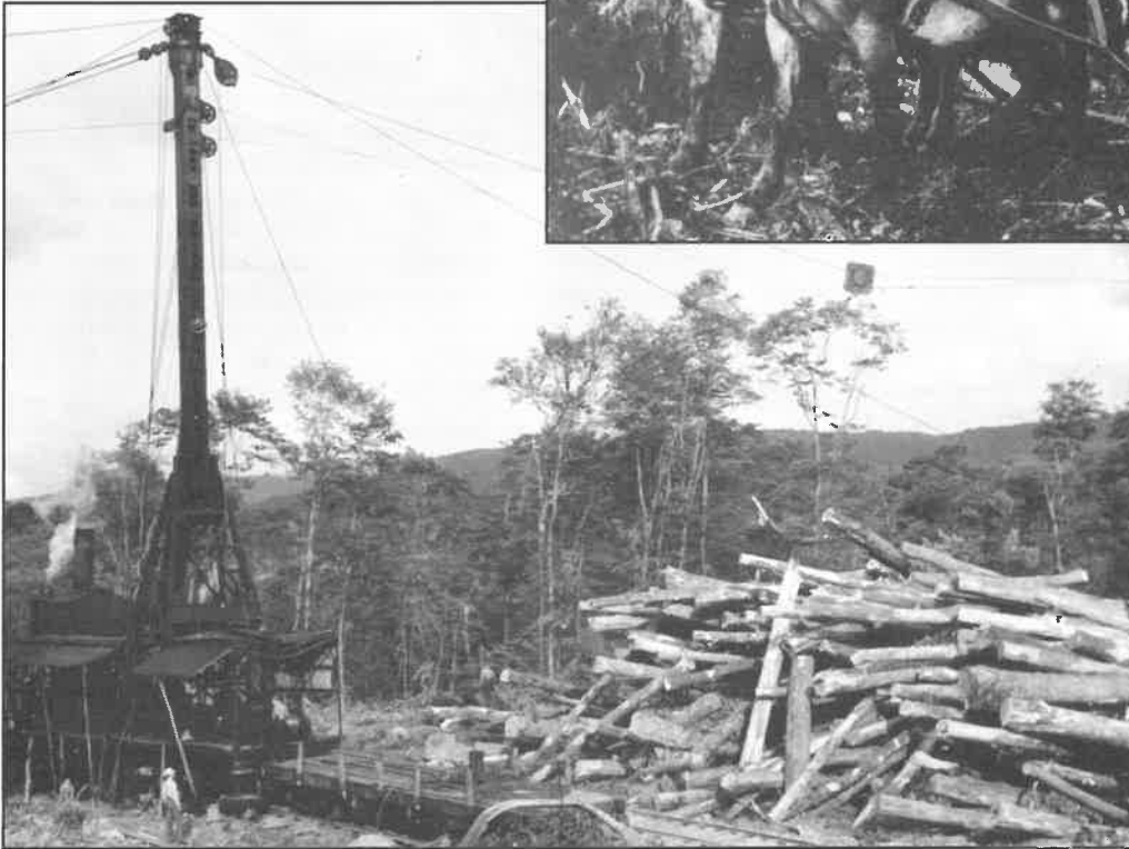
Opposite: This Barnhart loader used steam power to load logs. The company later designed modified loaders to handle tree-length logs. Photographer and date unknown.
