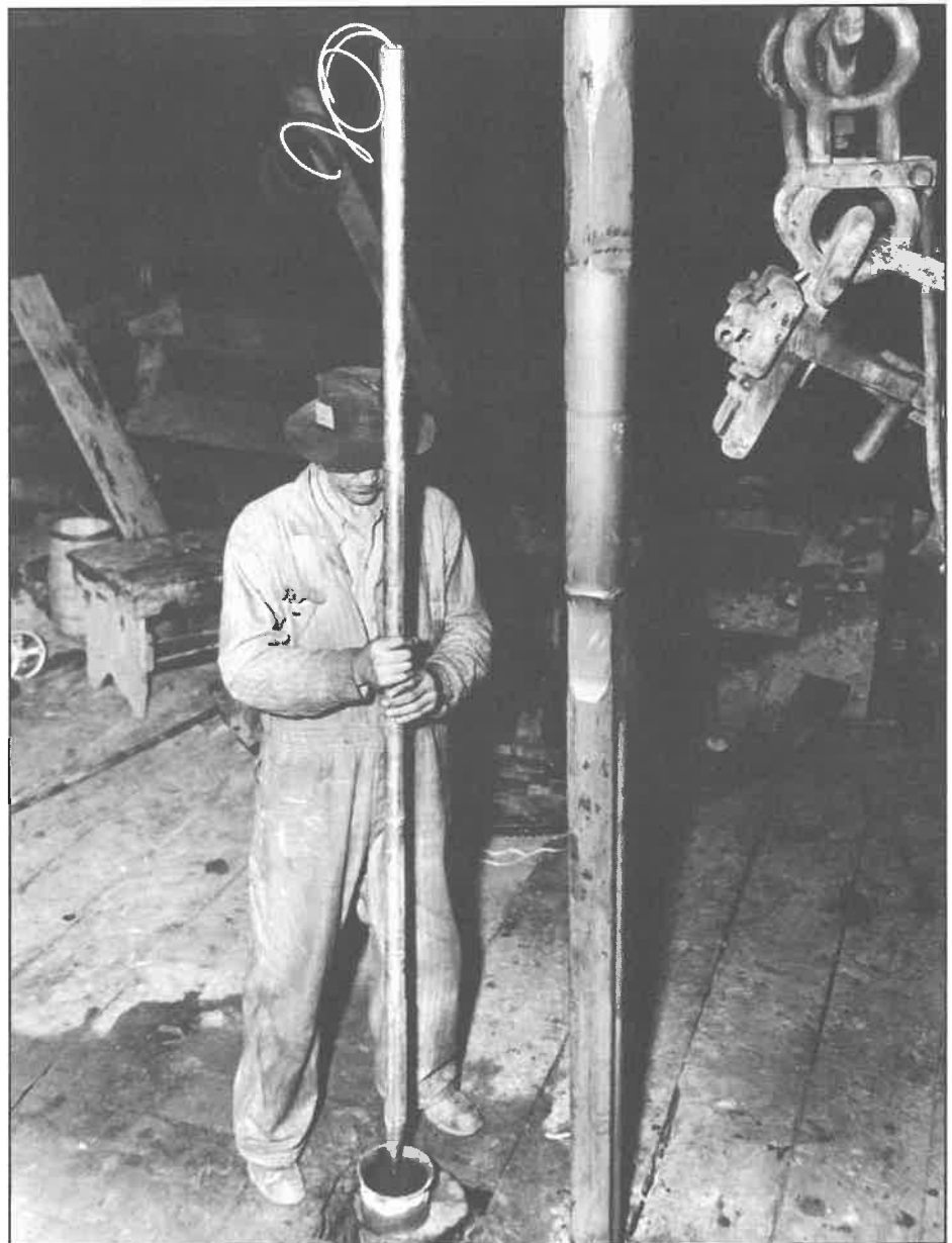
An Adkins employee prepares an explosive charge for a well on the Hatfield farm. Photographer unknown, 1949.
