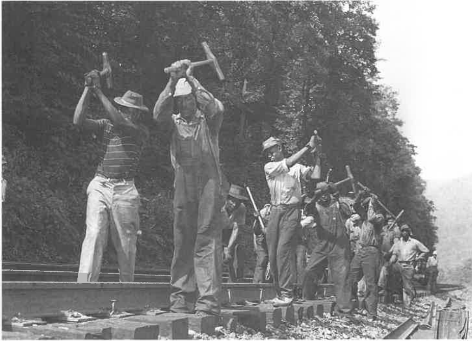
Track gang spikes down rails in the New River Gorge near Thayer, 1944. This was a common scene on railroads in the days before modern track-maintenance equipment. Photographer unknown, courtesy the C&O Historical Society.
