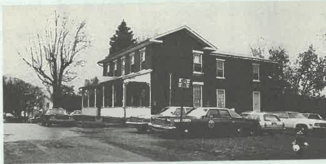
The old Ritchie County jail and sheriff's residence at about the time the Hinkles lived there. Photo by Dan Deibler, courtesy State Historic Preservation Unit.
