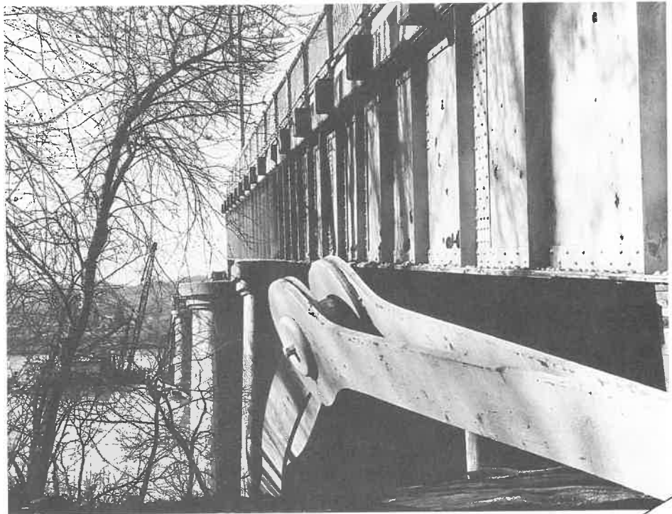
The bridge's unusual eyebar-chain construction was the key to its engineering and its collapse. The photograph shows one of the big eyebars after the crash, while the cutaway drawing shows a typical joint. The vertical element descends to support the bridge deck below. Photo by Herb Clagg, courtesy West Virginia State Archives; drawing courtesy National Transportation Safety Board.
