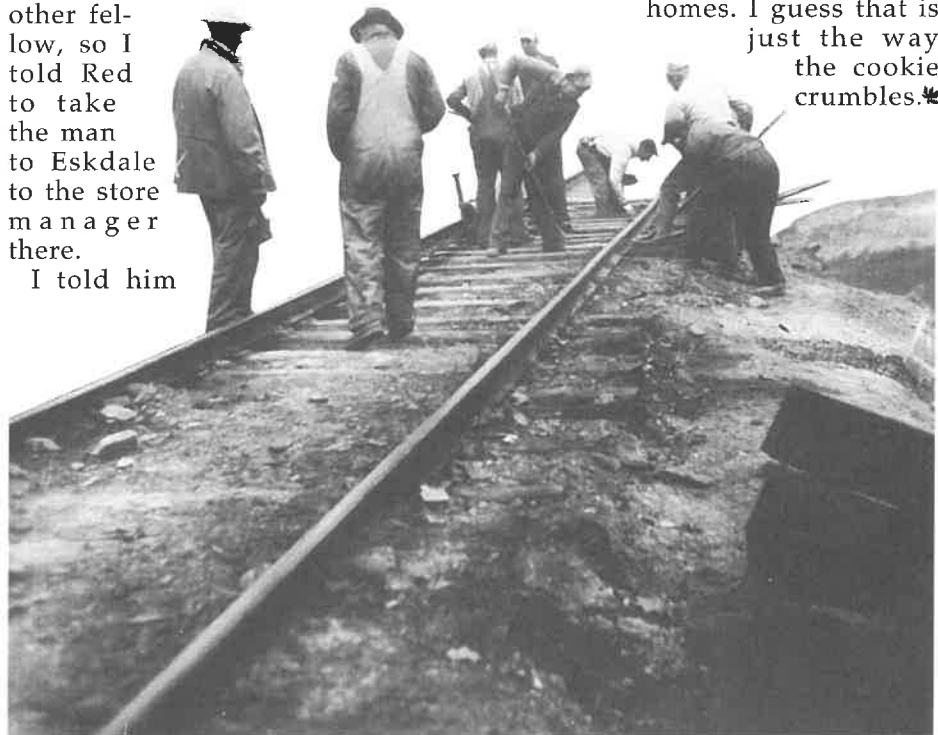
The conflict brought discouraging times to Widen. These men labor to repair strike damage to the coal-hauling railroad.
