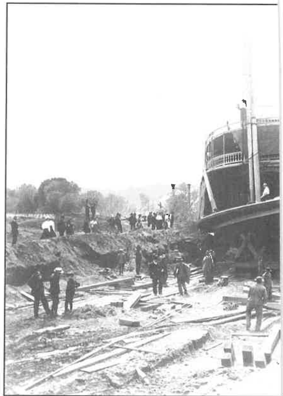
Once the big boat was braced, the idea was to ease it down the chute to the Ohio River. Photo by Captain Jesse P. Hughes, courtesy Public Library of Cincinnati and Hamilton County.
