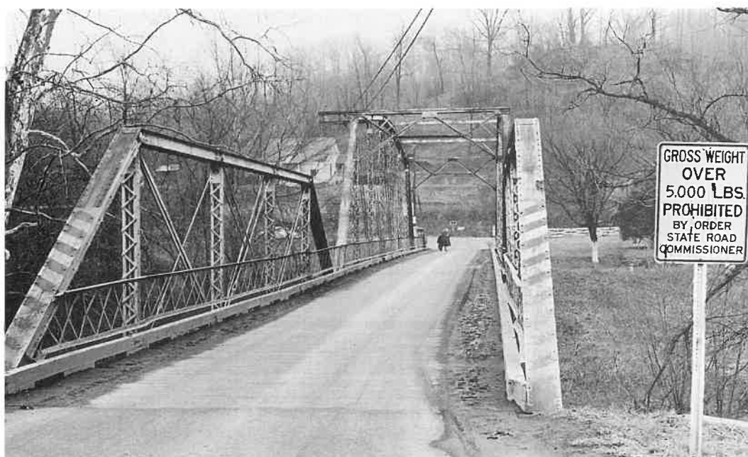
The bridge had been posted down to 5,000 pounds before refurbishing, a problem for school buses and other heavy vehicles. Photographer unknown, courtesy Huntington Herald-Dispatch .
