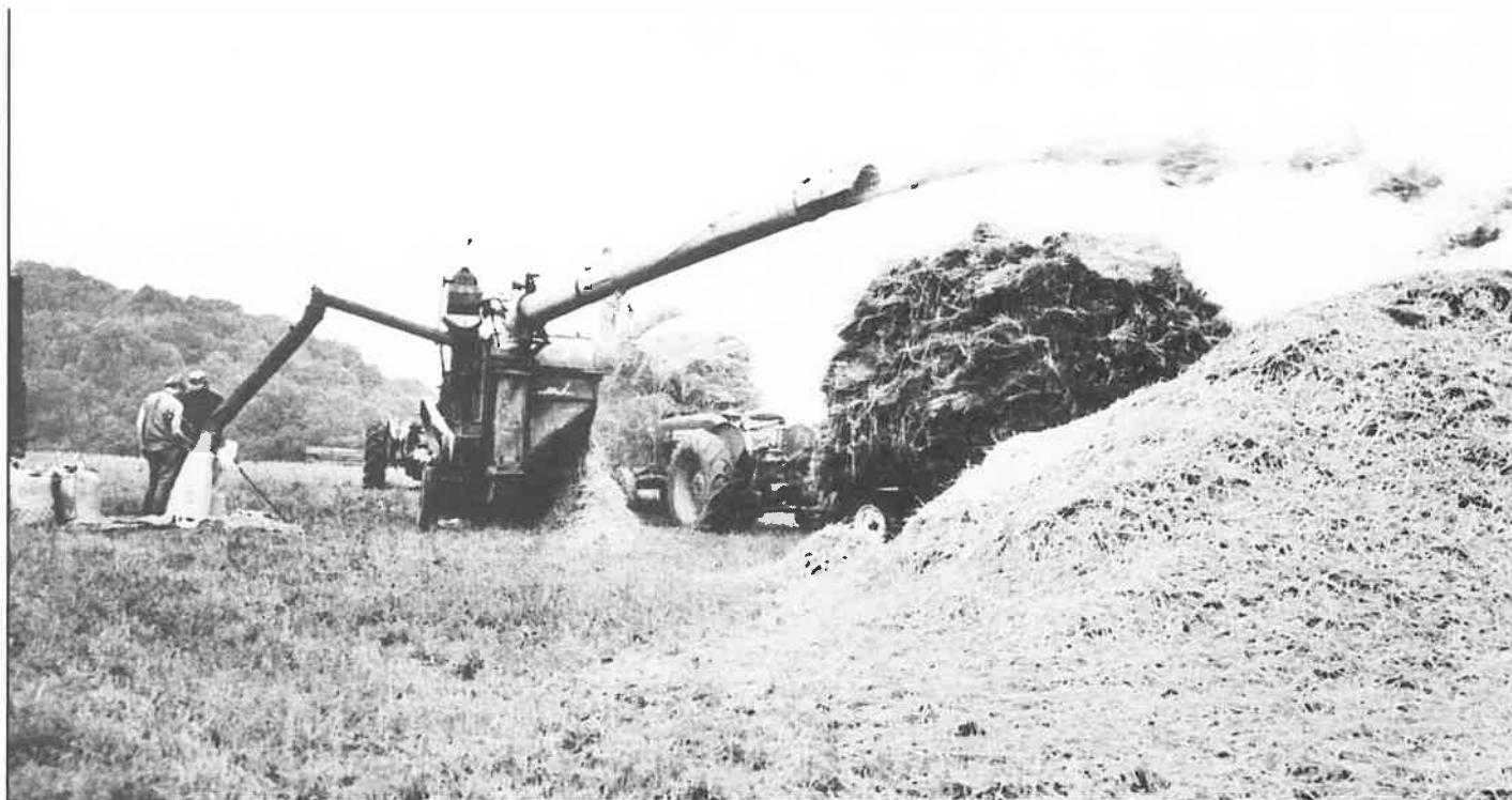
After threshing, the straw is blown out through a chute for later stacking. The threshed grain comes out the smaller chute on the left, where it is bagged. Photographer unknown.
