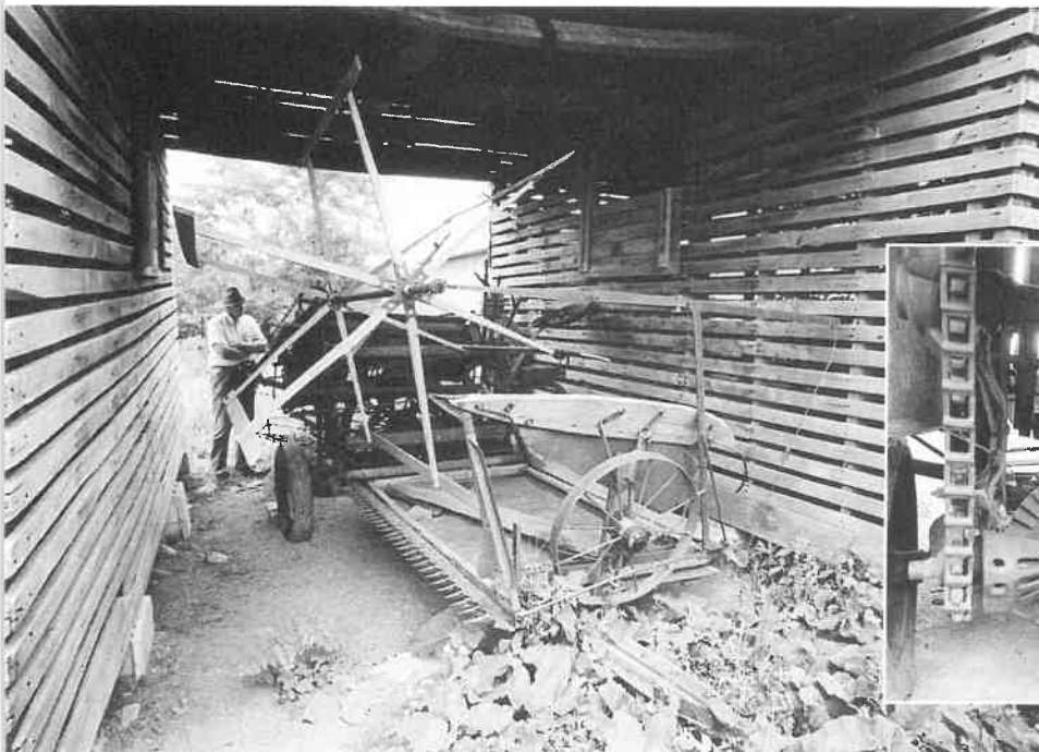
Author Gene Bailey inspects a reaper, or "buncher," stored between two corn cribs on Hugh Gooch's farm. This piece of harvesting equipment is pulled through the fields by draft horses or by a tractor, where it cuts and bundles stalks of grain.
