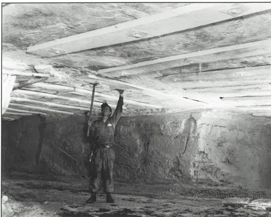
A mine foreman (or fireboss) checks (or sounds) the top. Note the white walls coated with limestone dust. Photographer and date unknown, courtesy of Jim Boner.
