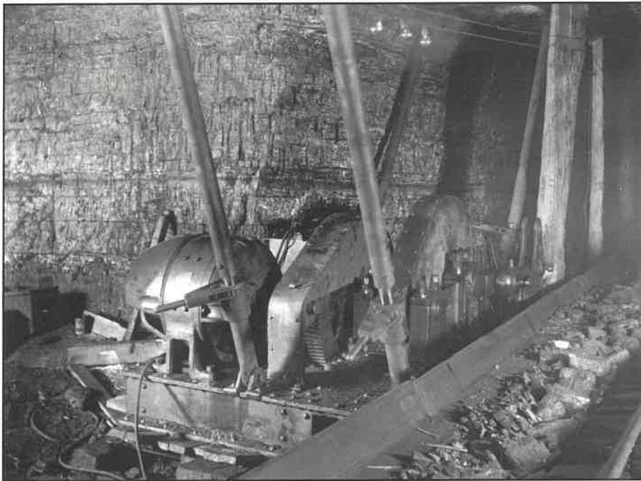
An Eickhoff conveyor drive unit in the mine at Gary No. 9. Behind this impressive machine is an even more impressive seam of coal, estimated to be about seven feet at this point. The Pocahontas Coalfields contained some of the richest coal reserves on earth. 1926 photograph from the Hornick Collection, courtesy of the Eastern Regional Coal Archives.
