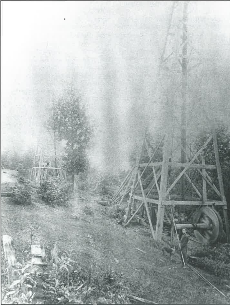
At its peak, Volcano was one of the most successful and productive oil towns in the country, thanks in part to W.C. Stile's innovative "endless cable" pumping system. This method allowed as many as 40 wells to be run by a single power station, requiring only one operator. Walter Taitt had the difficult job of keeping the system in operation, repairing the cable whenever it broke. Photograph taken in 1900, courtesy of West Virginia State Archives, WVSA hereafter.
