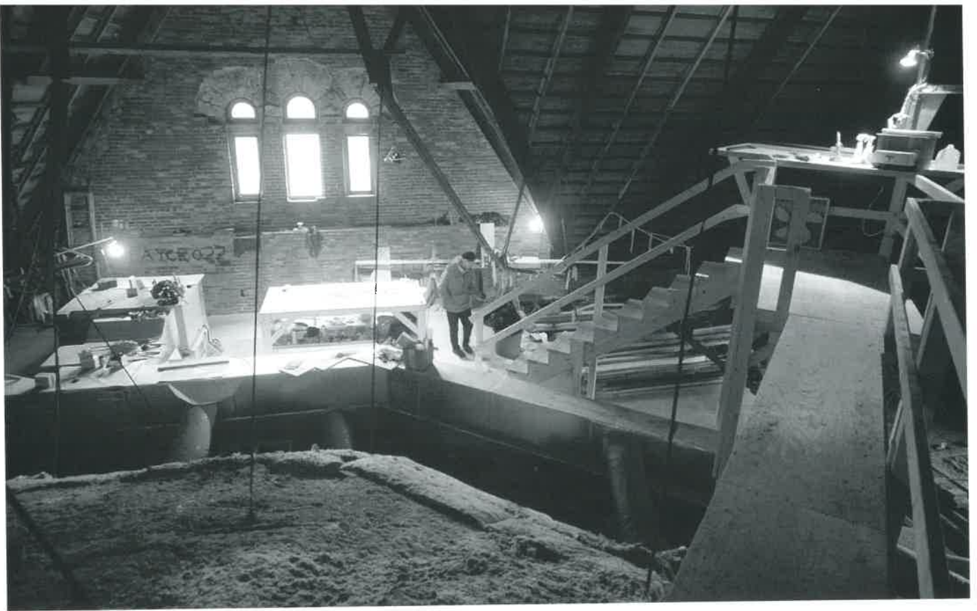
This elaborate temporary workshop was built above the courtroom for Grace and Joe to use during the dome restoration.
