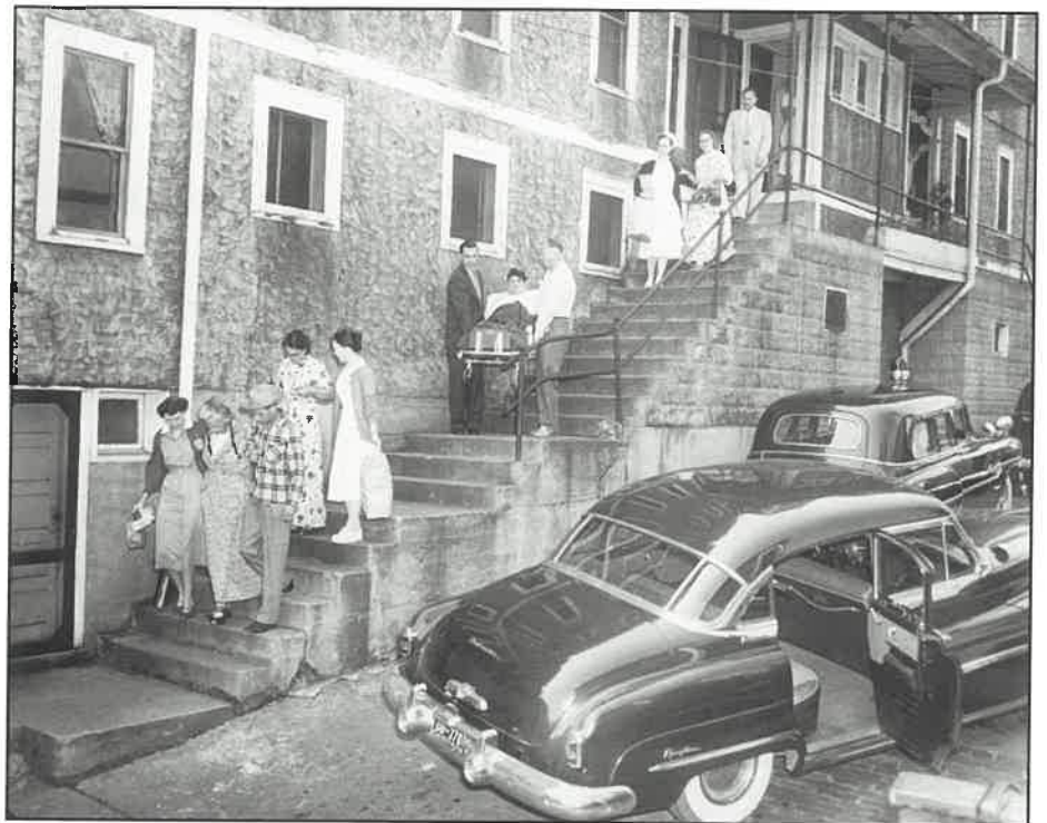
Steep terrain and the lack of an elevator at Sacred Heart Hospital meant that patients either walked or were carried in and out of the building, or from floor to floor. This photograph shows patients exiting the hospital in the 1950's.
