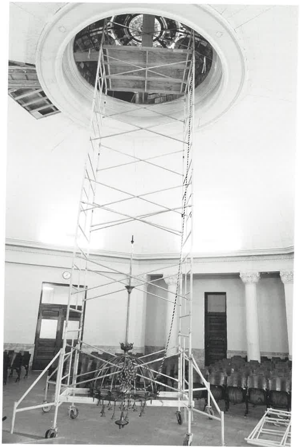
The courtroom of the Randolph County courthouse. This tall scaffold allows Grace and Joe access to the underside of the dome.
