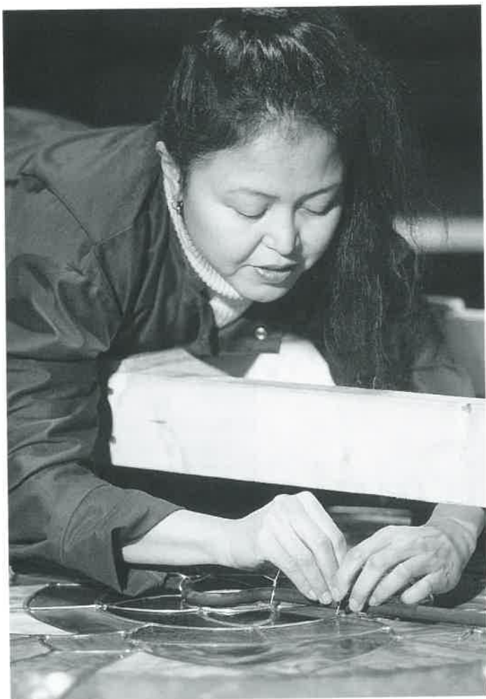
Grace Obana is an experienced stained glass artist who has learned to be cautious, especially when working in a precarious position, such as this. Here, she is stretched out on a board above the dome, 35-feet in the air, securing the centerpiece with small pieces of copper wire.
