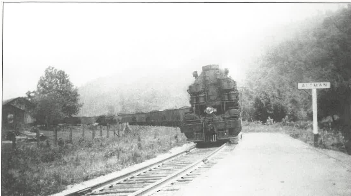
An empty C&O coal train approaches the Altman station in Boone County in 1947. Photograph by Warren Vance.
