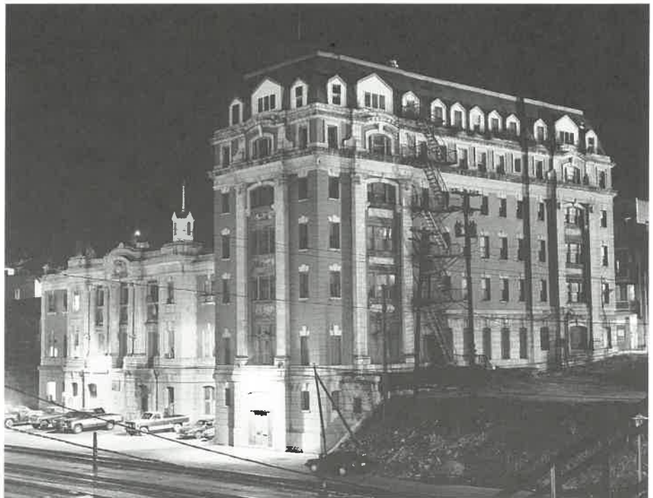
The B&O station and Willard Hotel at night. Both buildings are scheduled for renovation as part of a recent downtown revitalization effort in Grafton. Photograph 1997 by Jay Potter.
