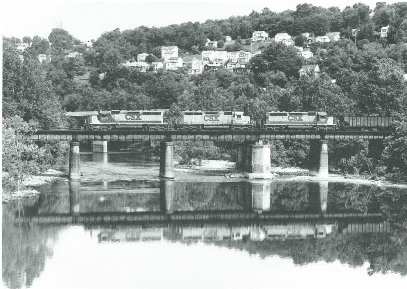
Three locomotives on an empty coal train are reflected in the water near the confluence of the Tygart Valley River and Three Fork Creek, with a Grafton residential neighborhood visible on the hillside in the distance on July 18, 1997.
