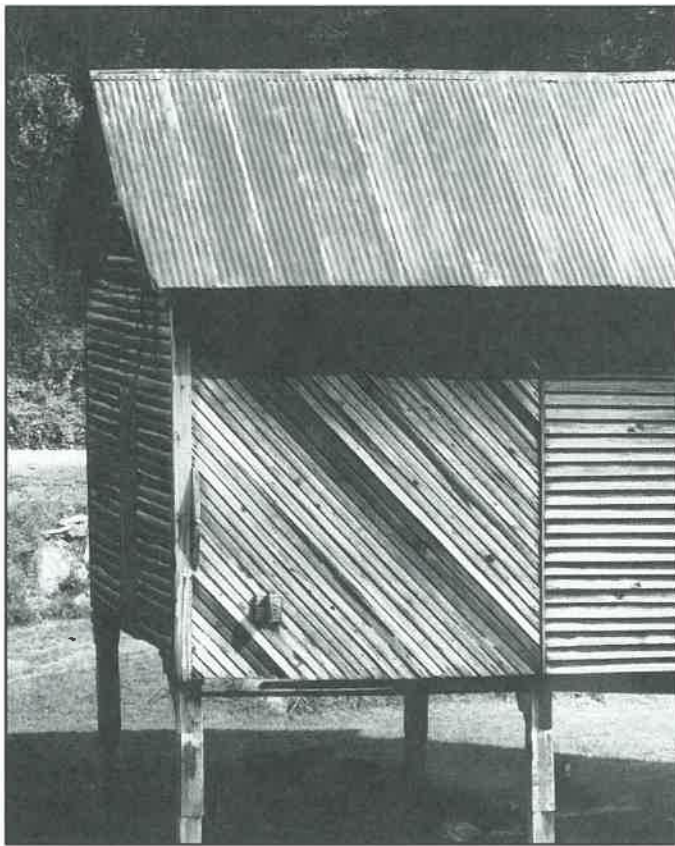
This innovative granary was built in 1900. It is raised on six-foot posts lined with tin to discourage climbing rodents. The sheltered area beneath the granary was used to store farm equipment, while the granary itself had chambers to store corn and wheat. Photographer and date unknown.
