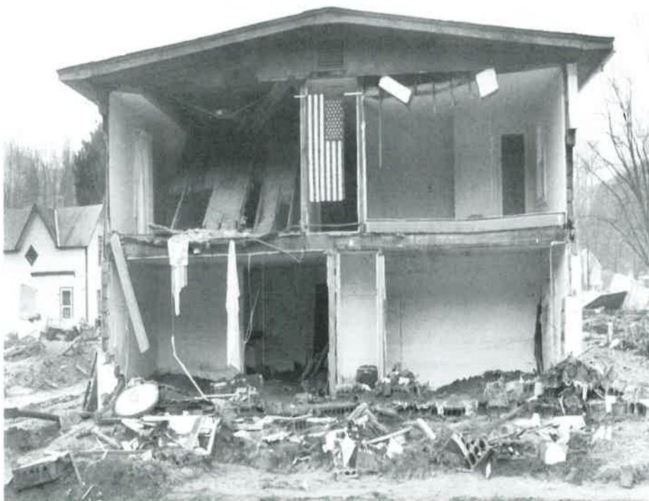
The Wilson Apartments on Pennsylvania Avenue in Parsons were among hundreds of buildings destroyed, damaged, or condemned due to the flood. More than 4,000 homes were destroyed statewide. This photograph was taken on November 14.
