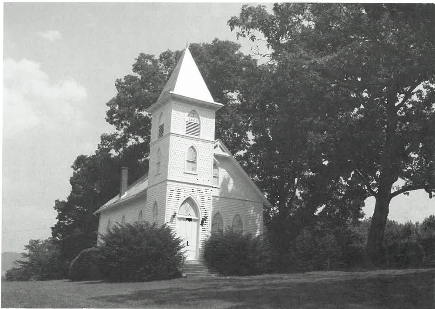
The Upper Tract Presbyterian Church in Pendleton County. Photograph by Michael Keller.
