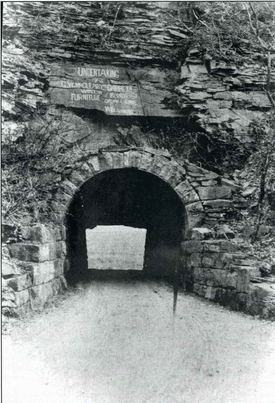
The Waugh Tunnel, one of two tunnels carved along this route in the 1830's, helped reduce the trip between Wellsburg and Bethany from 19 miles to seven. The tunnels were later widened to accommodate trolley traffic.
