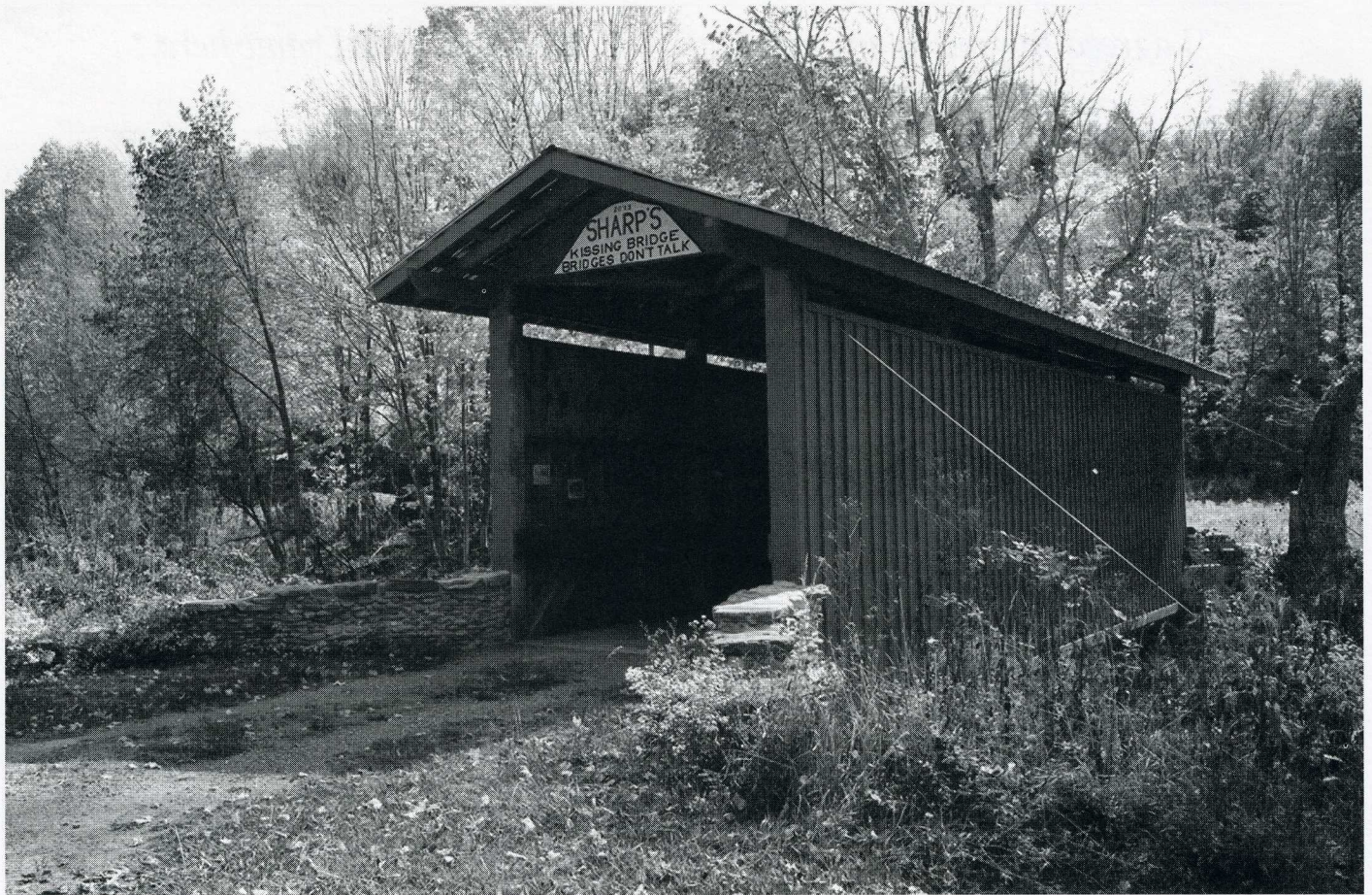
This 50-foot covered bridge was built in 2005 to honor Dave Sharp. It leads across the Big Spring Fork of the Elk River to a pasture and cemetery.
