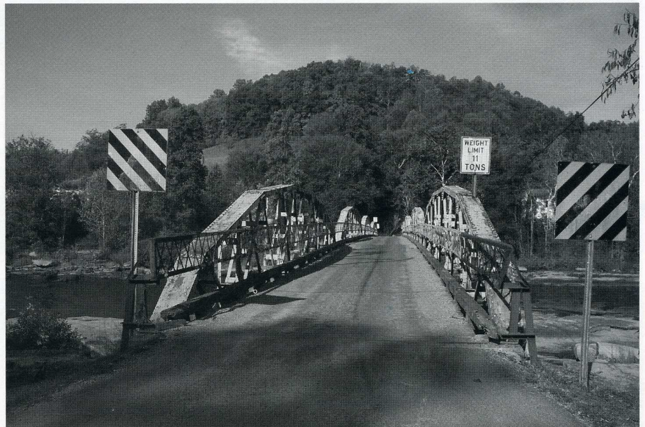
The Blue Bridge, built circa 1908, crosses the Tygart Valley River at Arden. Photograph by Richard S. Bailey.
