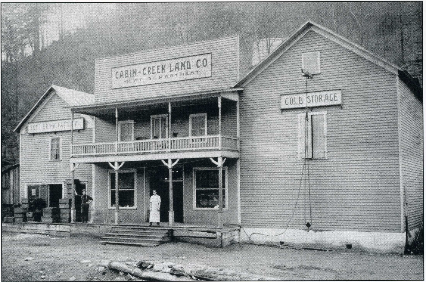
Original Decota store. Photograph courtesy of the West Virginia State Archives.
