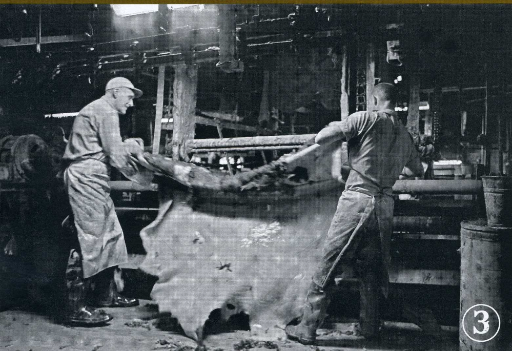
3) Ed Peck, at left, and an unidentified coworker operate a hairing machine to strip hair from hides. All of the work to prepare hides for actual tanning takes place in the beam house, so called because of the complex array of I-beams hung from the ceiling.
