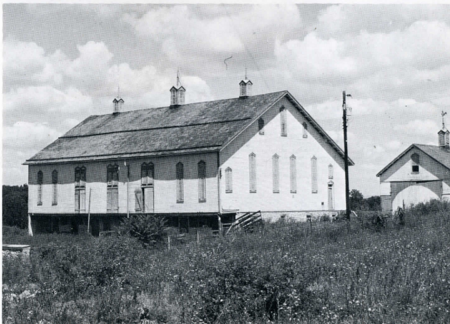
Below. The Kunkel Barn-Berkeley County. This is the best remaining model of the large German-Pennsylvania Bank barn. Built in 1910, it is 100 feet long by 60 feet wide, with limestone foundation and German siding.
