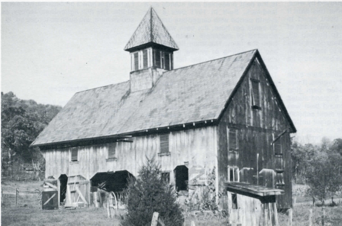
Below. Harrison County-1870s. The Boggess Barn with slate gable roof and large cupola with chestnut wood walls.
