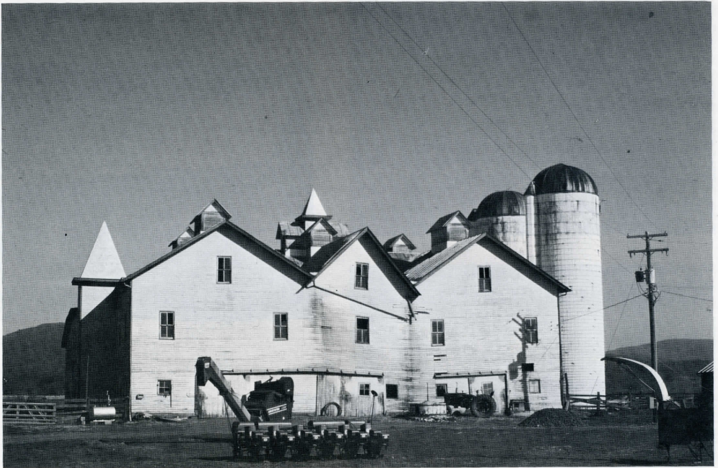
The Leatherman Barn-Hardy County. Built in 1904 of German siding and set on locust posts, this is three barns in one. Note church-like entrance on side and twelve cupolas.
