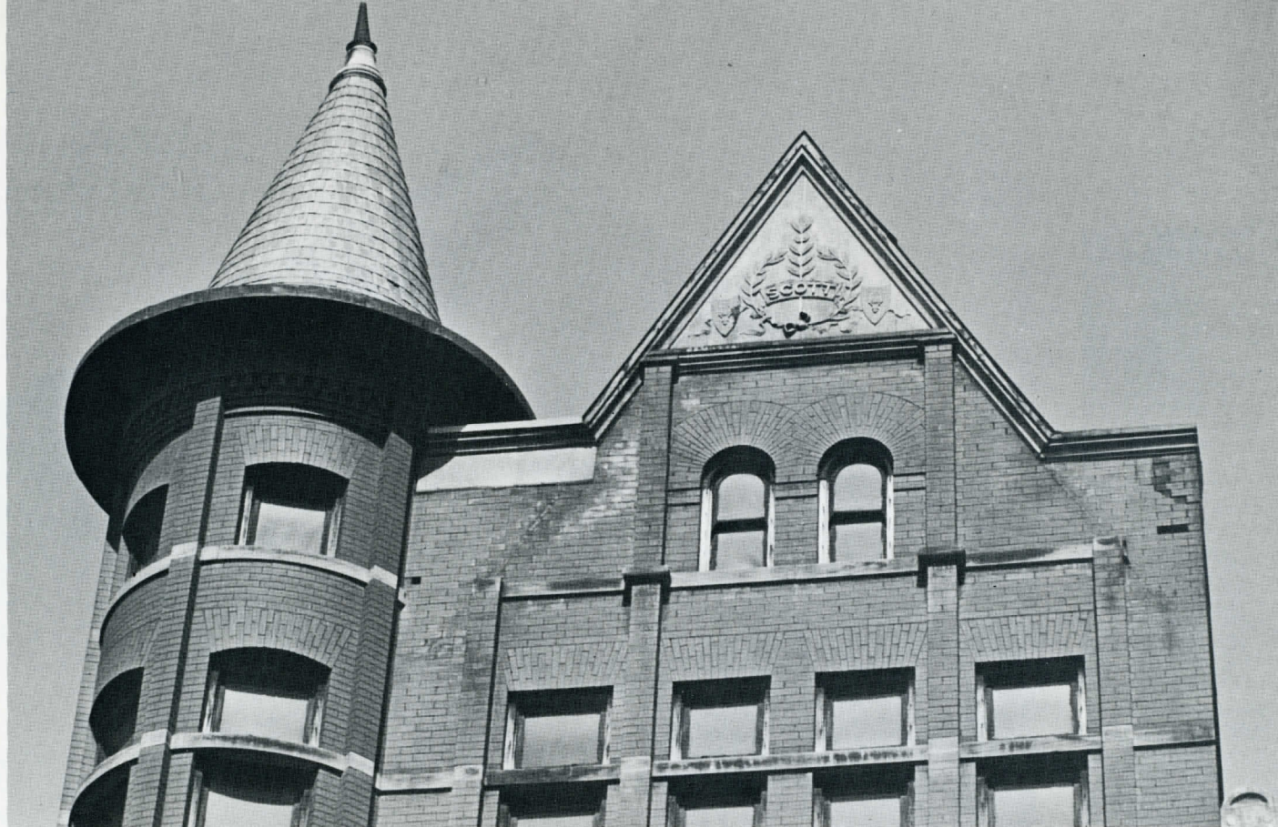
Conical cap, jack arches, and gable plate on the Scott Building at 227 Capitol Street.
