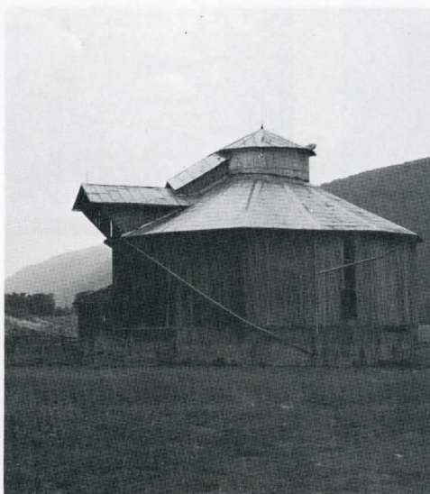
Top. Doddridge County-1870s. All wood barn with boarded up timbers and A-framed gable roof.
