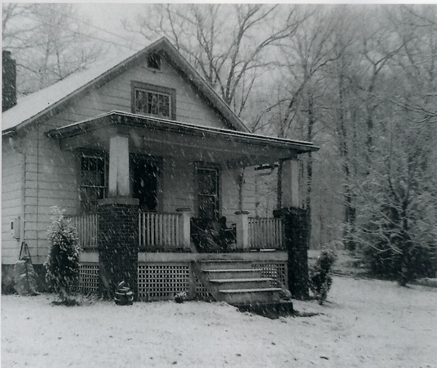
The Lemley house is seen here during a snowstorm, probably in the winter of 1959-60. Today, the entrance to the West Virginia Botanic Garden and the upper parking lot for the garden are to the right of where the house stood.
