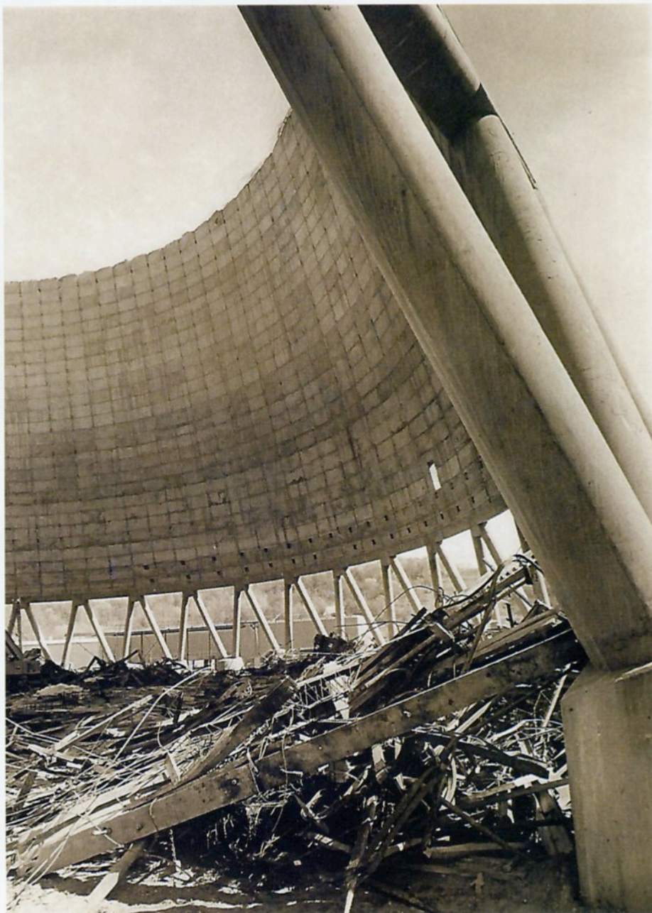
The twisted remains of scaffolding are scattered beneath the half-finished cooling tower at Willow Island, April 27, 1978. Photo by John Klein, courtesy of James E. Casto and the Huntington Herald-Dispatch .
