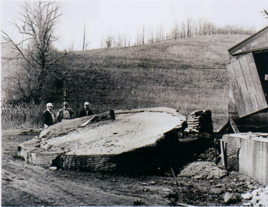
One of the explosions blew this 26-ton cap from the Mod's Run air shaft of No. 9. Courtesy of the WVSA, Department of Mines Collection.
