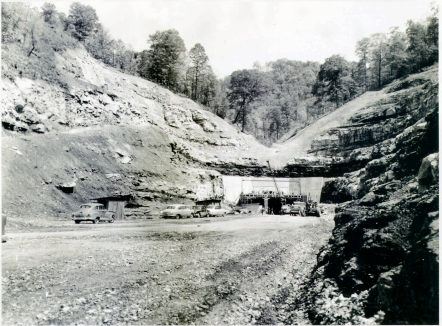
The 88-mile West Virginia Turnpike required the construction of 110 bridges and the moving of 30 million cubic yards of earth. One of the biggest challenges was the two-lane Memorial Tunnel, connecting Dawes and Standard. It took two years to build and claimed the lives of five workers. Courtesy of the West Virginia State Archives (WVSA).
