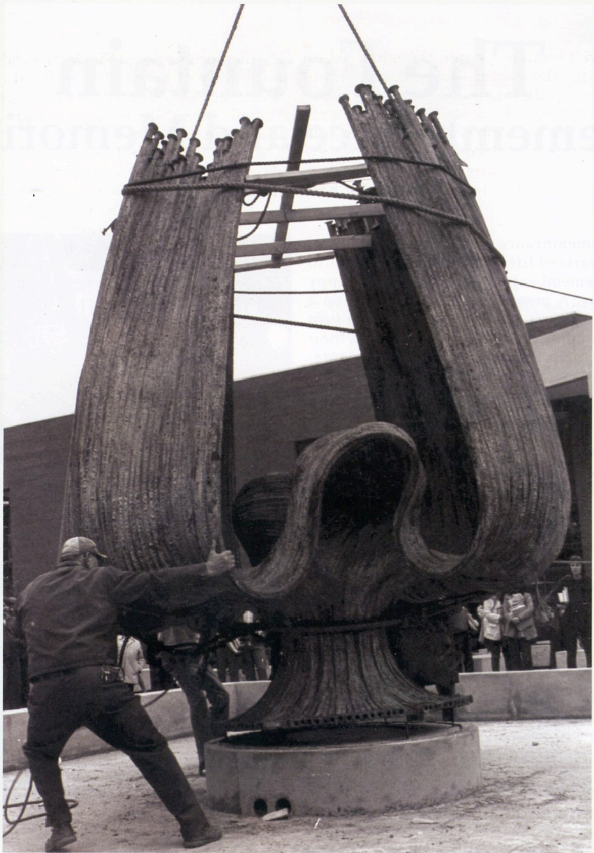
Workers lower the 6,500-pound Marshall Memorial Fountain into place, 1972. Courtesy of Marshall University Special Collections.
