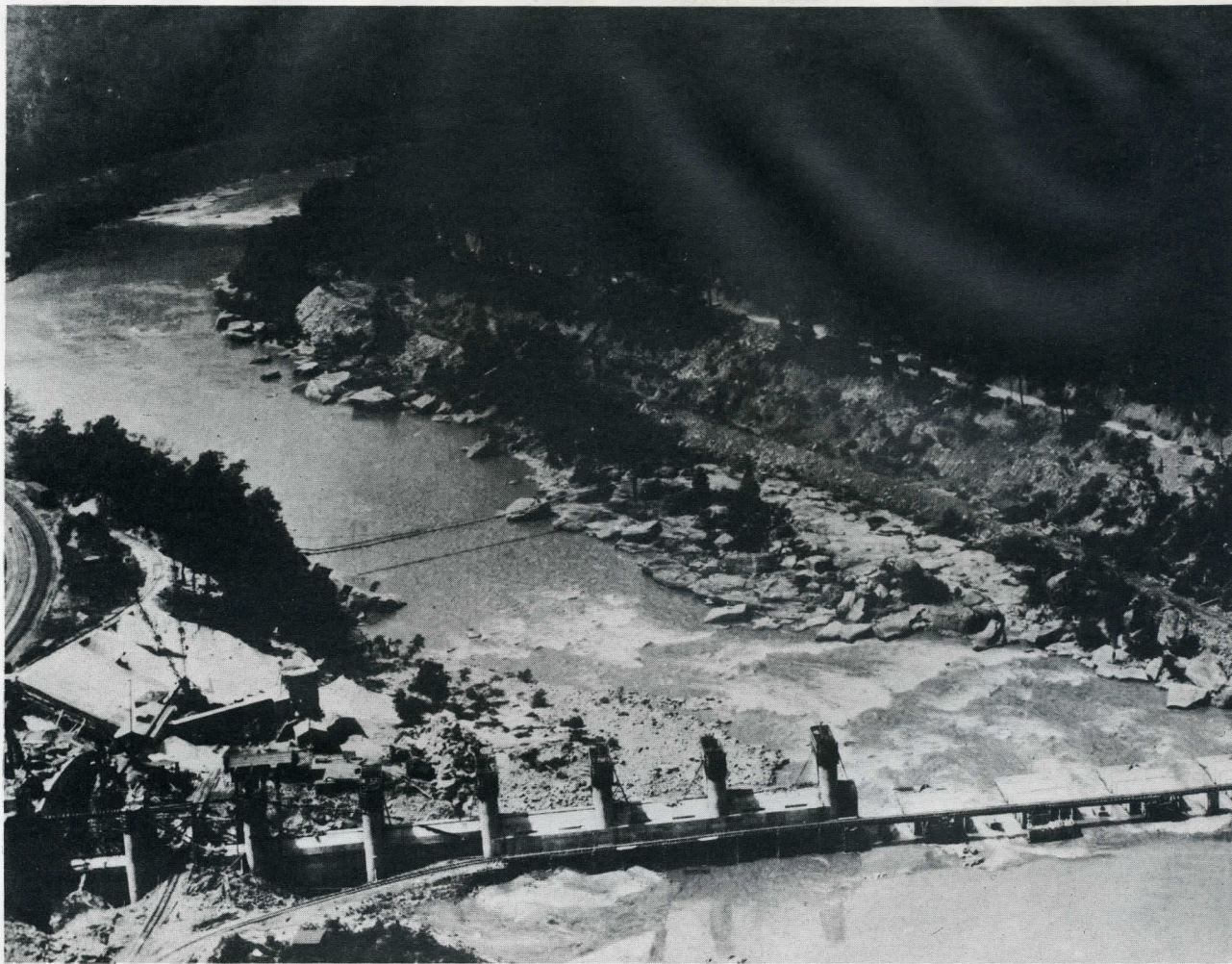
Construction of the Hawk's Nest Dam. The tunnel (for which we were unable to locate construction photographs) began here, carrying water to a hydroelectric station near Gauley Bridge. Photographer unknown, courtesy West Virginia Collection.
