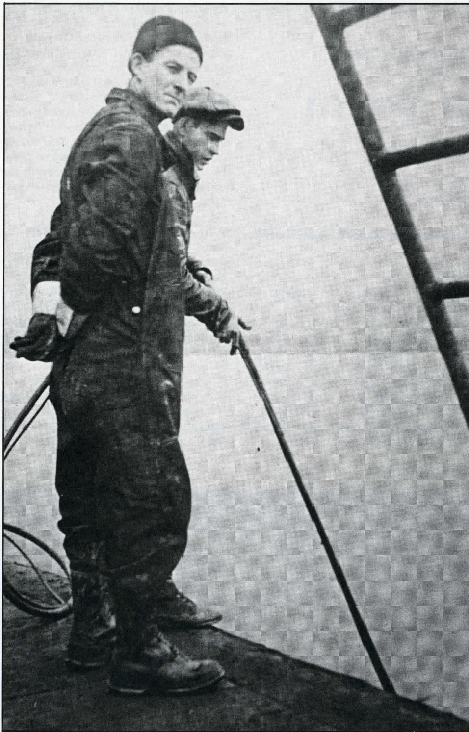
Diver's helpers, or tenders, had charge of the diver's safety underwater, watching the pump and seeing after his hose and rope lifeline. It was "pretty much of a responsibility," as Mr. McGuffin says. Date and photographer unknown.
