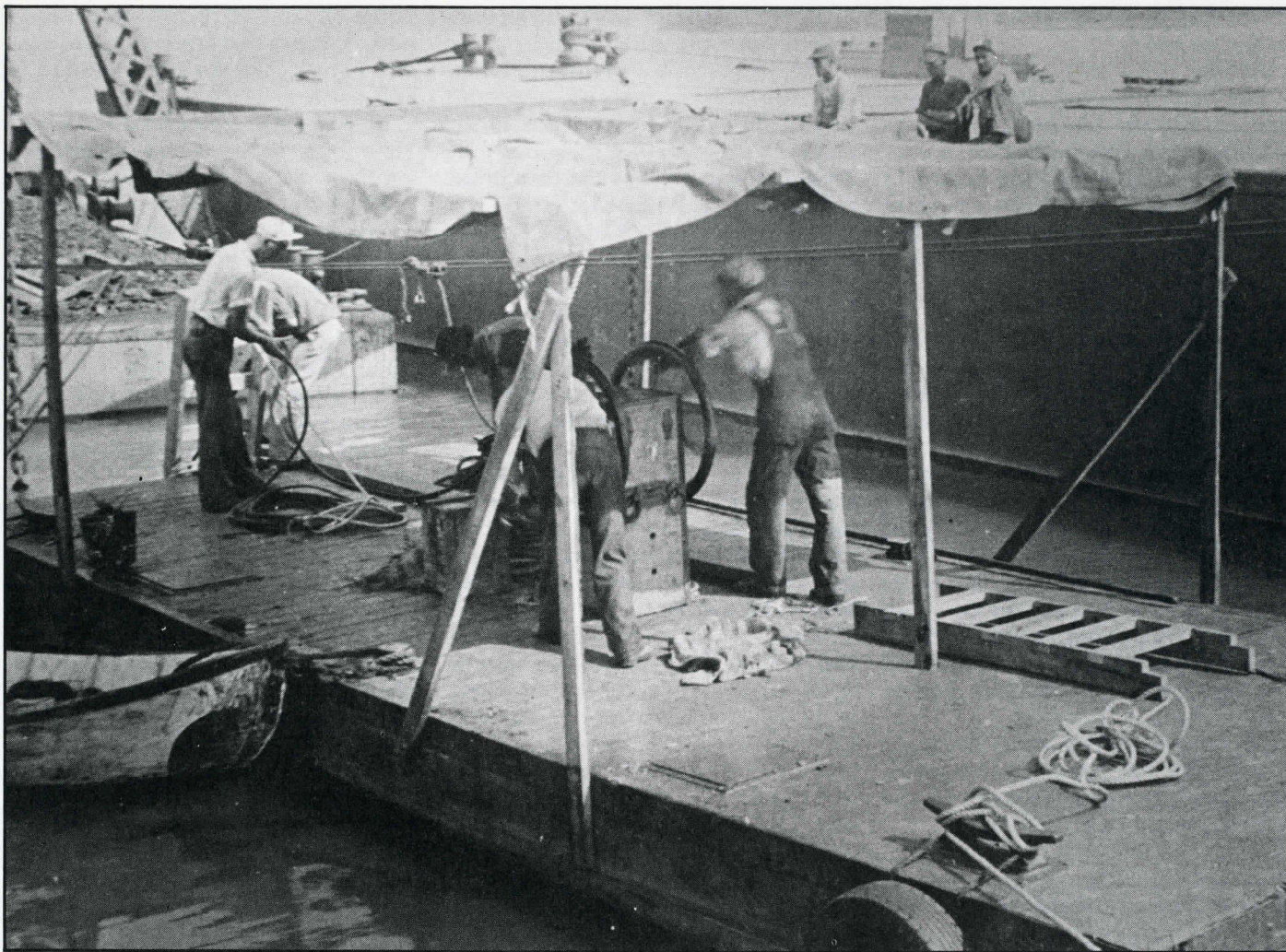
Pump helpers manning a two-handed air pump for the diver below. The tender, partly visible at the front of the float, bends over to hold the hose and lifeline. Date and photographer unknown.
